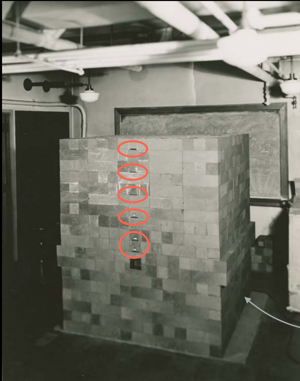
Test pile at Columbia
