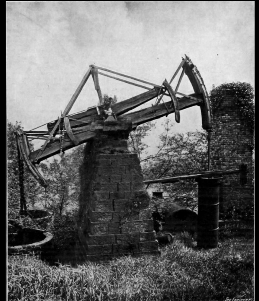
"Fairbottom Bobs" at a coal mine in Lancashire, England (operating 1760-1827)
