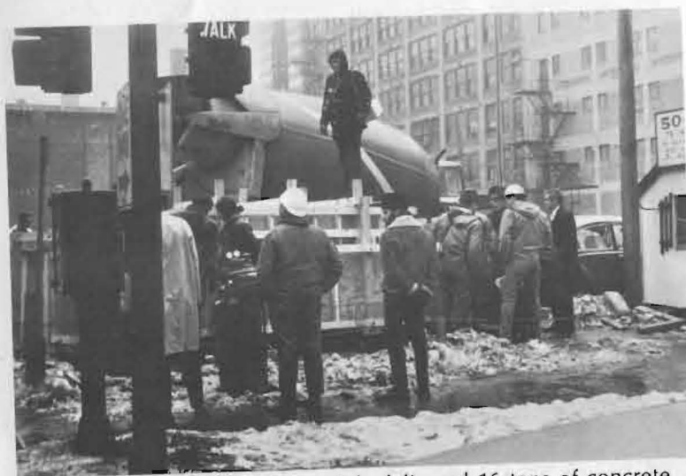
Later that morning Vulcan Materials delivered 16 tons of concrete. Which was poured and shoveled into the form.
