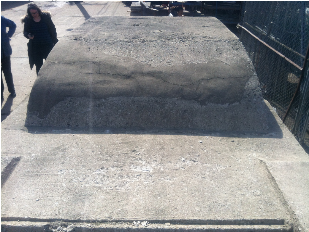
Figure 7: Concrete Traffic , 1970, in storage at Methods & Materials, Chicago IL, January 2012, showing the state of the concrete patching in 2012, the same enclosed in red in previous image
