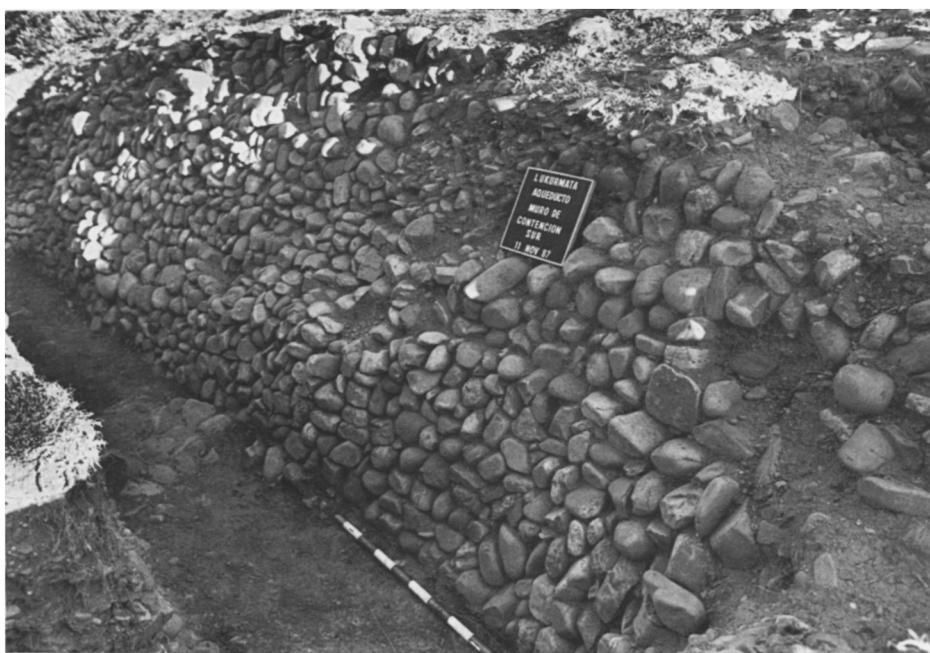
Figure 7. Aqueduct terraced retention walls.
