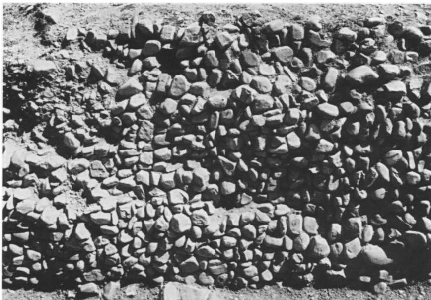
Figure 6. Detail of basal construction of the Lukurmata aqueduct.
